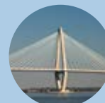
Wire breaks monitoring of bridges
